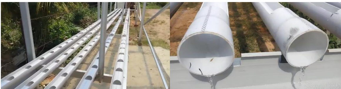
Gambar 6. Instalasi Pipa 300 Lobang
